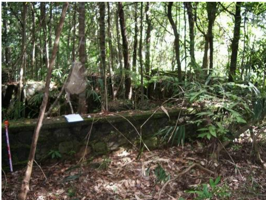
Figure C- 72 CR HS7, Strele, Lot 40, northern end of main structure
