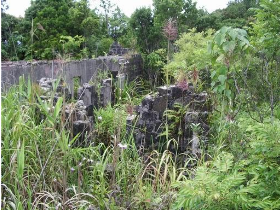
Figure C- 79 ER HS6 Jouffrey lots 80-81 Looking across site from northwest corner.
