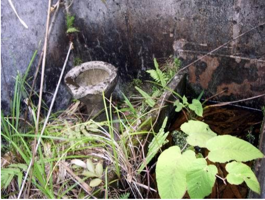
Figure C- 84 WR HS4, Lot 76. Bathroom on southeast corner
