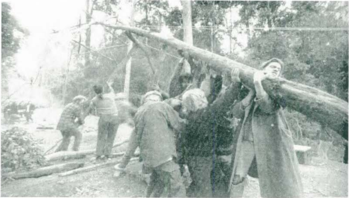
Figure 64: Erection of tripod.
