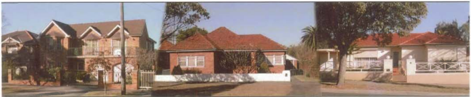
Figure 4-15: Strathfield – Security screens and shutters on residential buildings
