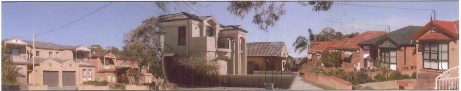
Figure 4-24: Kingsgrove – More recent redevelopments
