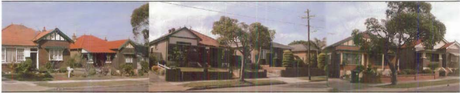
Figure 4-18: Roselands – Well maintained older style houses
