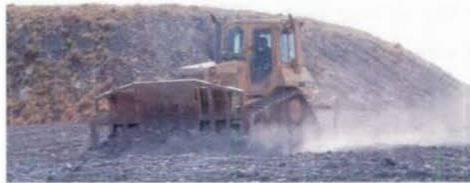
Figure 3.5: Machinery used for rock raking after ripping of overburden.
