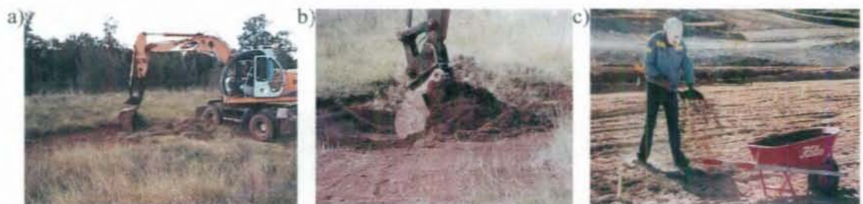
Figure 7.6: (a) Fresh topsoil collection by backhoe, (b) fresh topsoil bucket load and (c) manual spreading of fresh topsoil on plots (all at Cheshunt mine).
