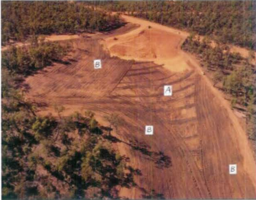
Figure 8.3: (A) Fresh topsoil applied in strips and (B) after the topsoil has been graded out at an Alcoa bauxite mine in Western Australia (Photo courtesy of Carl Grant). It should be noted however, that the rehabilitation objective in Alcoa bauxite mining is to return land to native ecosystems.
