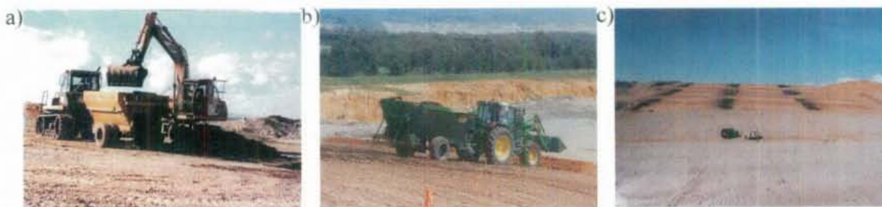
Figure 7.4: (a) Biosolids being put into the spreader, (b) spreading of biosolids on a rehabilitation site and (c) rehabilitated area following spreading (all at Cheshunt mine).
