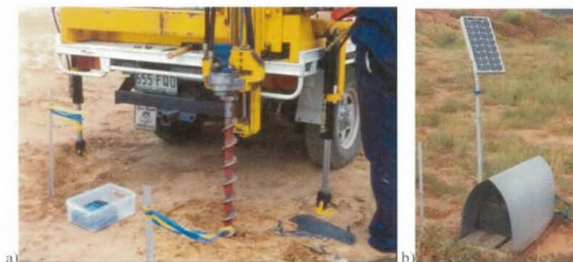
Figure 5.12: (a) Close up of auger drilling a hole for the data logger in a 6 m stockpile and (b) data logger location at the 6 m stockpile at Bengalla mine.
