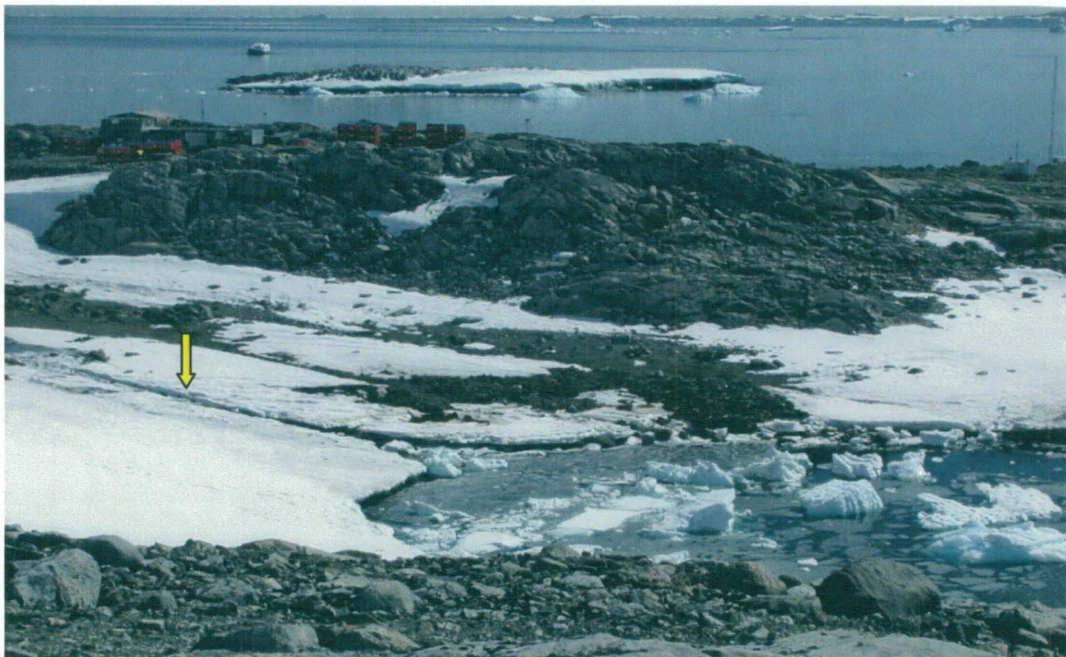
Figure 2.2.1. Brown Bay showing Thalla Valley tip site in 2002 showing channel dug to divert melt water from contaminated tip bed.
