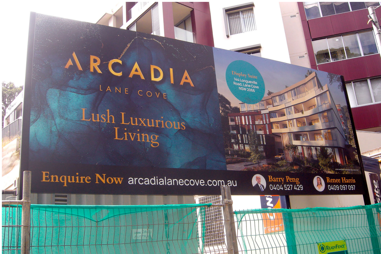
Figure 3. A boutique apartment block under construction in Lane Cove advertised as ‘Lush, Luxurious Living’.
