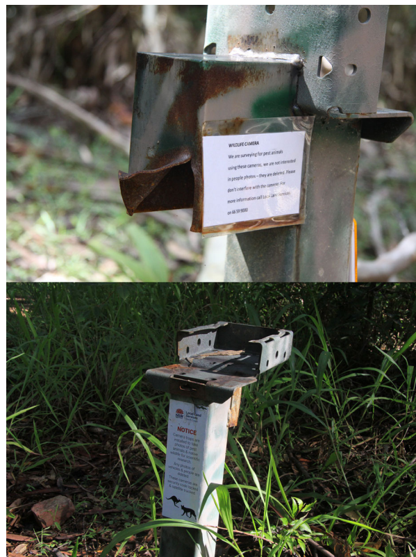
Figure 2. Security posts showing the modes of entry used by thieves to steal camera traps.
