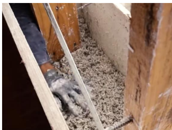
Hand packing in hemp house construction
