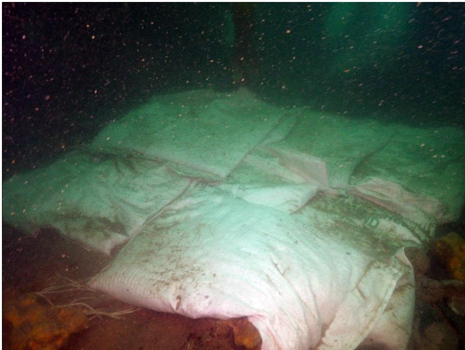
The final stage of the in-situ procedure over the excavated area
