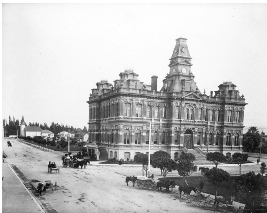
City Hall, San Jose, date unknown. Permission given by Catherine Mills, Curator, Research Library and Archives, History San Jose.
