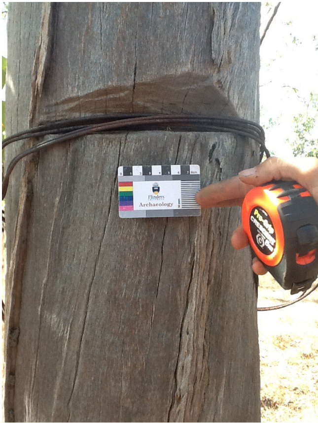
Figure 13. Typical post at Clayhole Yard 1, showing horizontal mark is only wide enough to support the wire for the horizontal rails.
