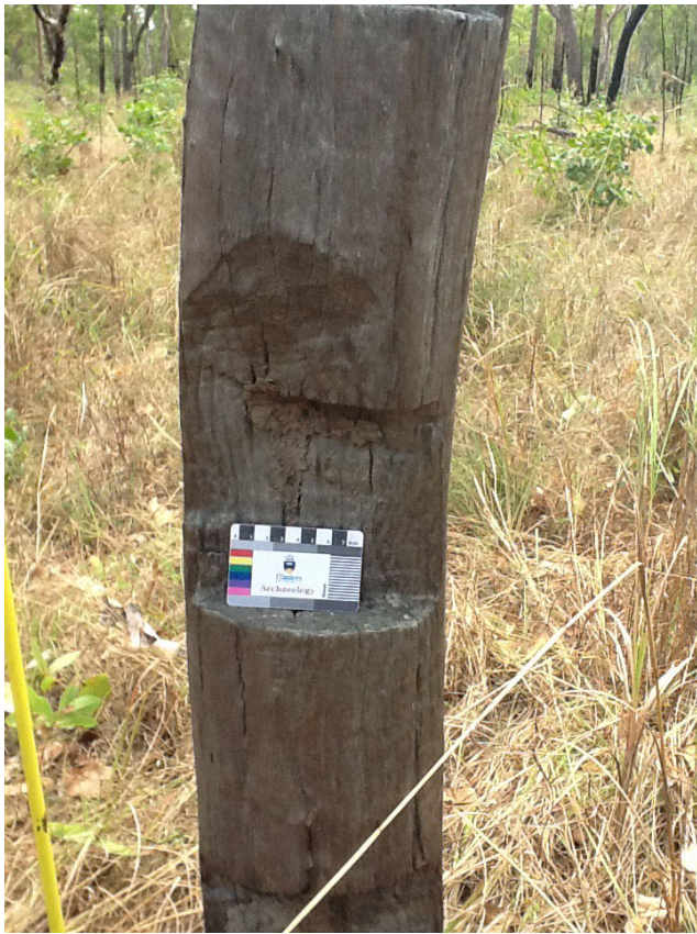
Figure 9. Billycan Yard 1, showing saw marks at the bottom of the fencing post and axe marks at the top.
