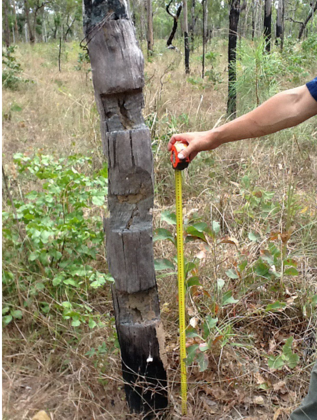
Figure 10. Billycan Yard 1, showing three horizontal saw marks and a bored hole for attaching a top rail at the top of the post.
