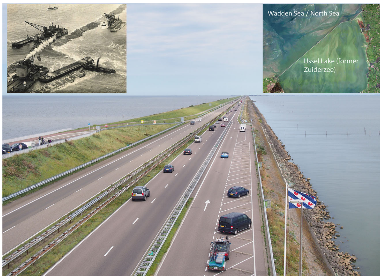
Figure 2. The 32km-long closure dam Afsluitdijk , separating the North Sea and Wadden Sea (left) from the IJssel lake (former Zuiderzee). Top left: the closure of the final gap of the dam in AD 1932 (Y.T. van Popta).
