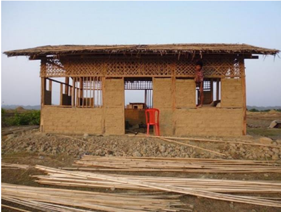
Figure 9-6 NEED TECC, Mrauk-U, Rakhine State (source: NEED, 12 September 2016).
