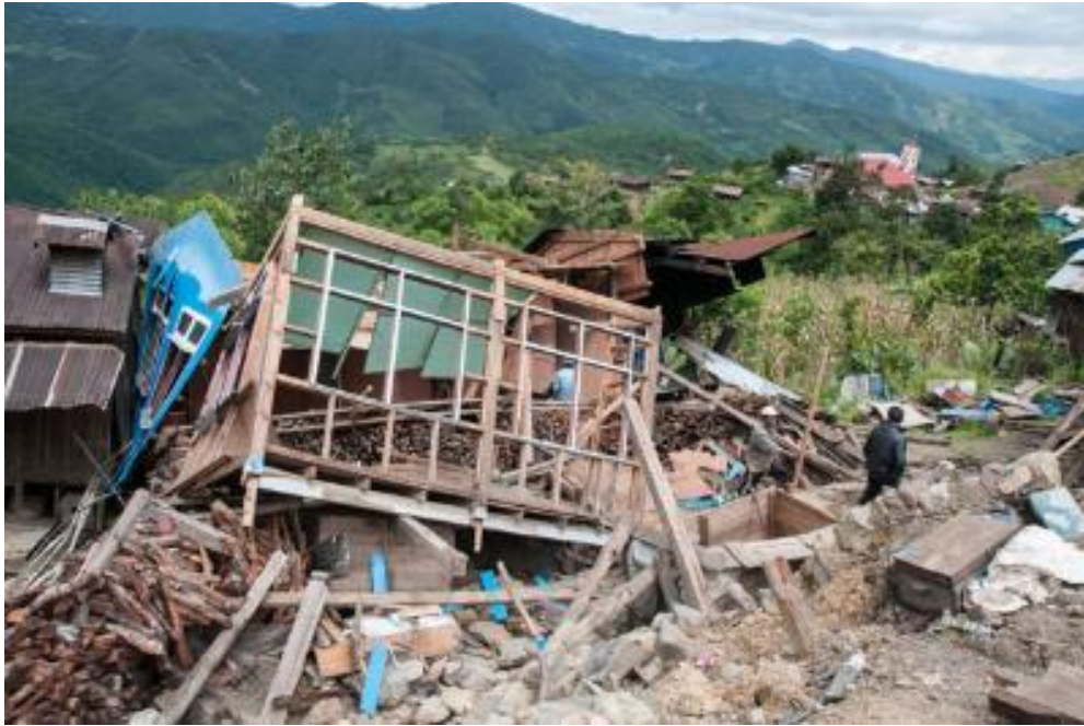
Figure 5-14 Houses destroyed by landslides Chin State, July 2015 (source: S8).
