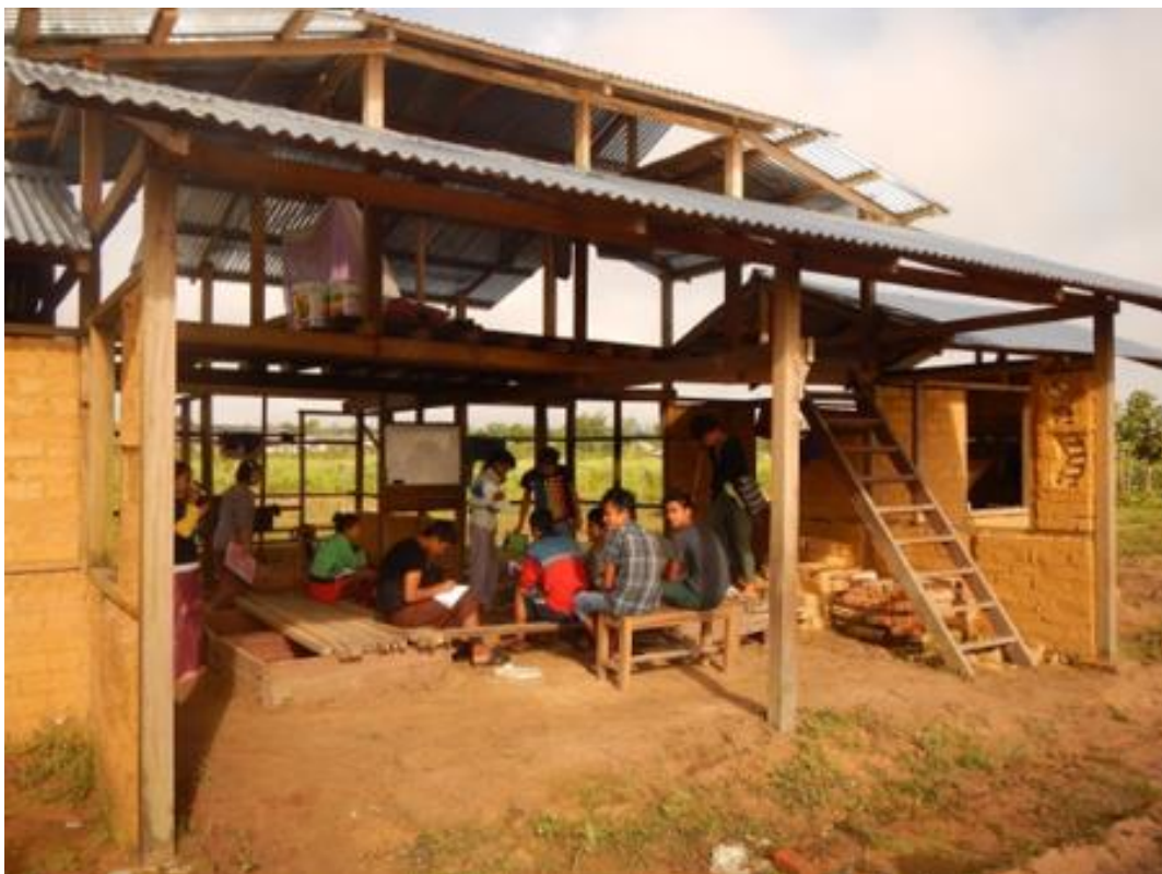
Figure 6-5 Schoolhouse on NEED Eco-Farm, December 2013.
