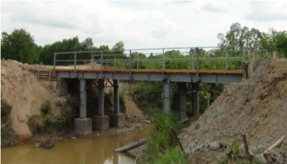
Figure 6-10 New bridge to NEED Farm, May 2014 (source: Ko Than Shwe).
