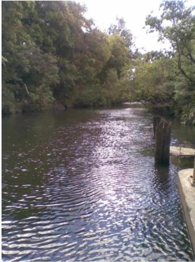
Figure 3.10 Dingo Creek at Belbourie Bridge (Looking downstream)
