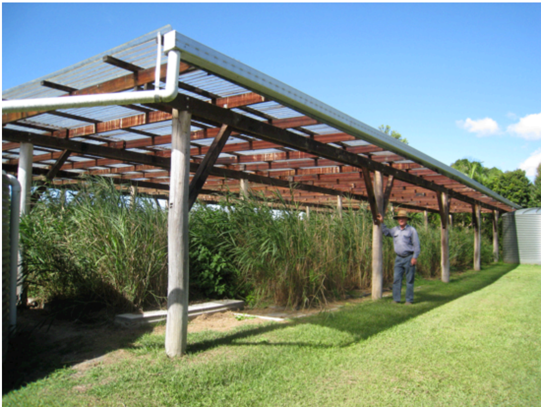
Ken Ohlson with the reed bed roof cover constructed by the Year11 students.
