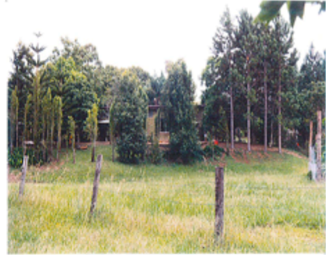
EXISTING BARN STRUCTURE
