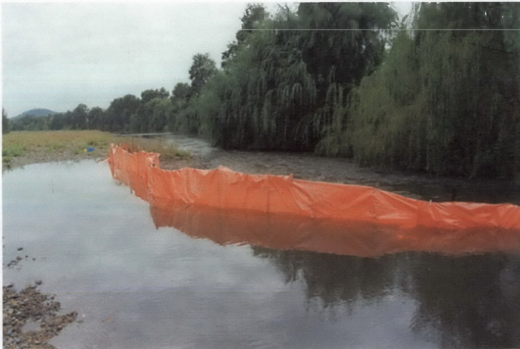
Figure 6.4. Looking downstream at Moses Crossing with the flow deflection fence in place.
