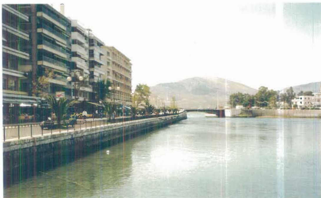
Fig. 1: The Euripos narrows and the swingbridge at Khalkis
