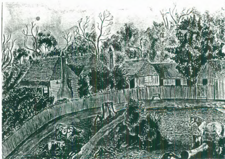
LINDESAY HOMESTEAD, 1877, a complex of slab and weatherboard structures, all with shingled roofs, (hipped except for the store on the extreme right.) The lefthand weatherboard building is apparently the most recent, being added in front of an earlier slab structure which may then have become a detached kitchen. Painting by Miss C. E. McDouall, 1877, copy by Mr. B. Ingles by courtesy of Nandewar Historical Society.
