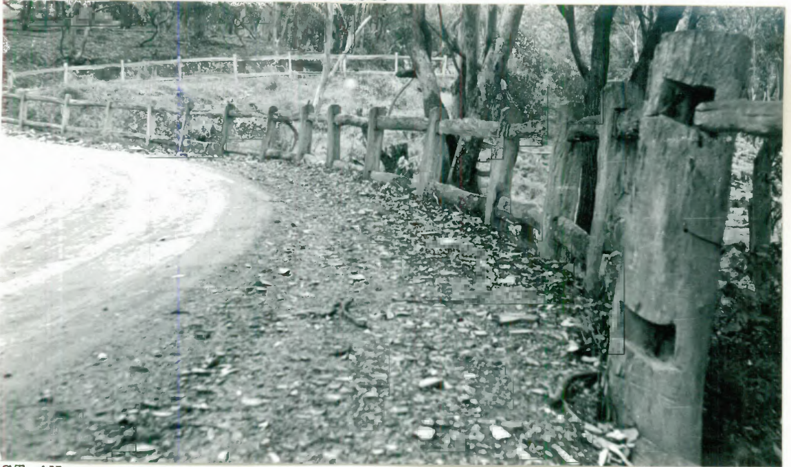
POST-AND-RAIL FENCE bordering the road between Sofala and Hill End. William Cox built similar fences along the more hazardous sections of his Blue Mountains road, 1814-1815. Photo.: L. G., 3 Sept., 1969.
